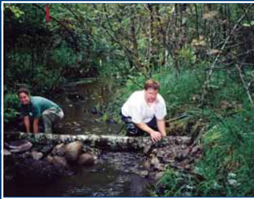
BCAF staff installing a digger log on Naas Brook, a small tributary within the Mushamush River watershed, Lunenburg County.
