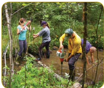
Crew hard at work installing a digger log.
