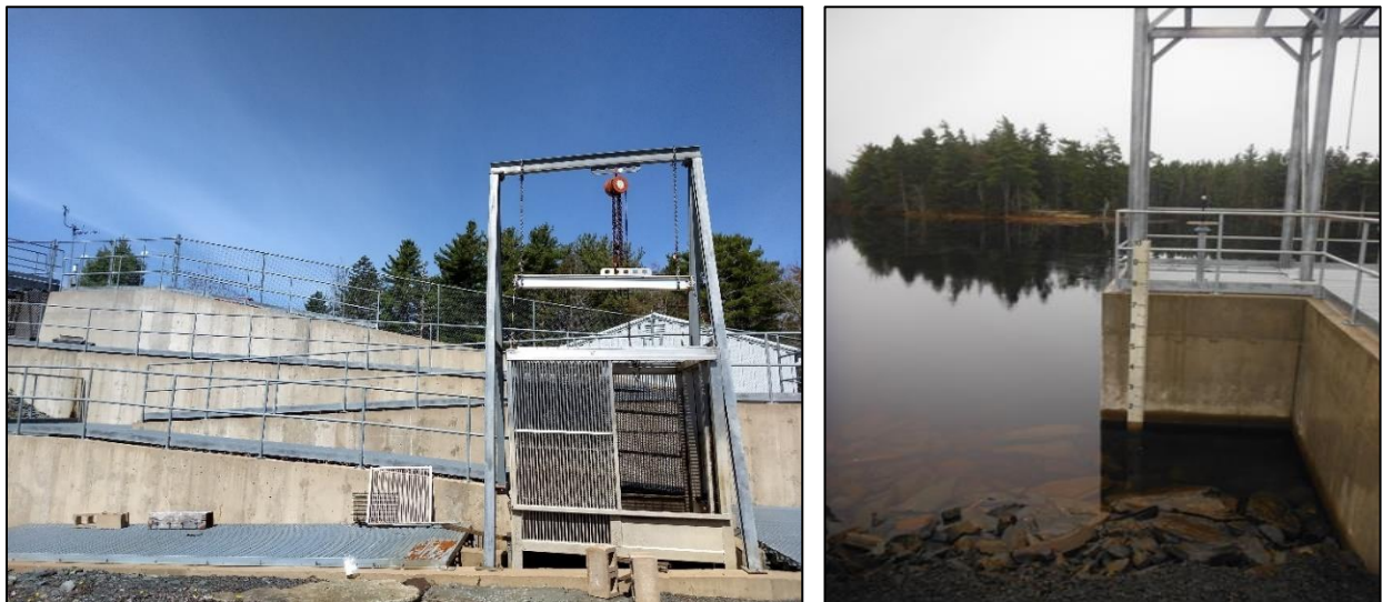
Figure 3. Left: Hebb Dam Fish Passage Facility trap lifted out of the fishway with door open. Right: Hebb Dam lake level gauge by fishway exit.
