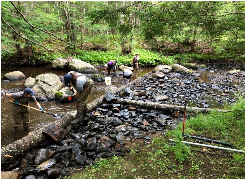
Figure 18. Photo showing a large digger log and deflector combination being installed on Zwicker Brook during the 2022 season.
