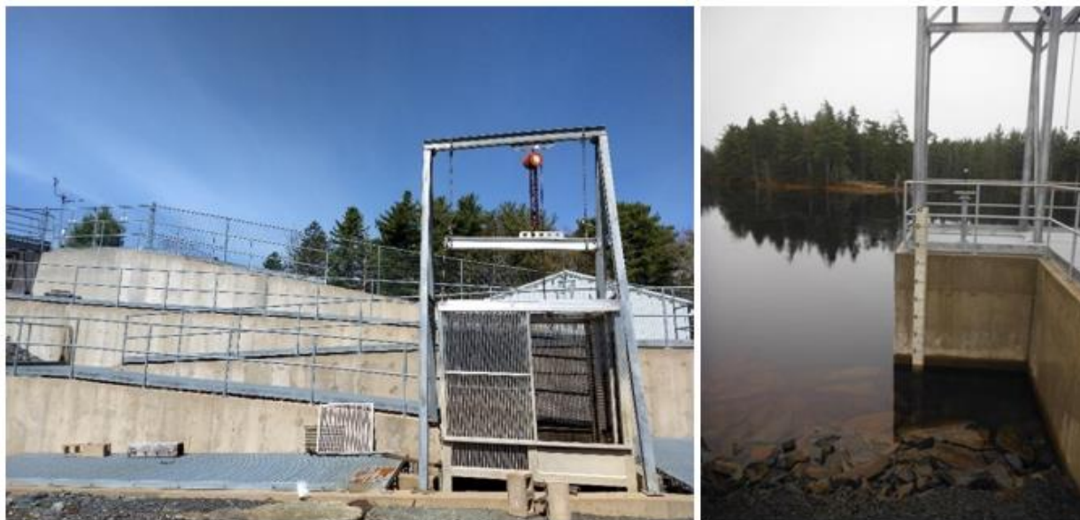
Figure 2. Left - Hebb Dam Fish Passage Trap lifted out of passage with door open. Right - Hebb Dam water level gauge near fishway exit.
