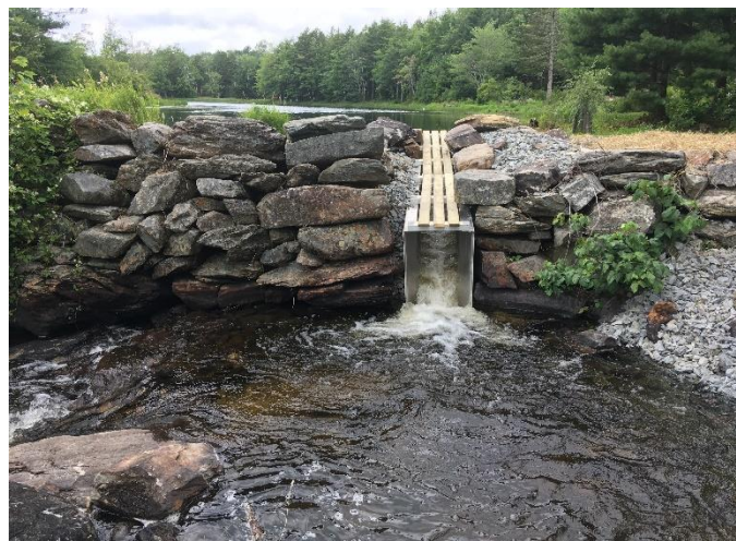
Figure 7. Photos from above (left) and below (right) the fishway at Crousetown Dam after it was installed in 2018.
