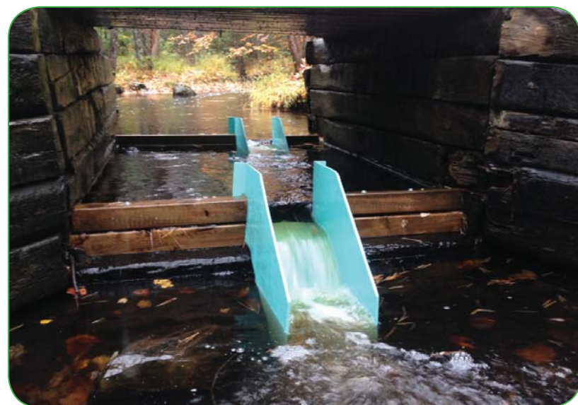
Restoring fish passage through a barrier culvert on Hebb Brook.
