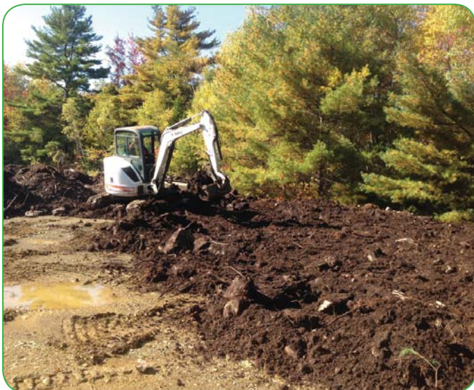
Organic soils being spread at the Wildcat Shale Pit Project site.
