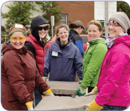
Volunteers remove broken segments of unused pavement in Ontario.
