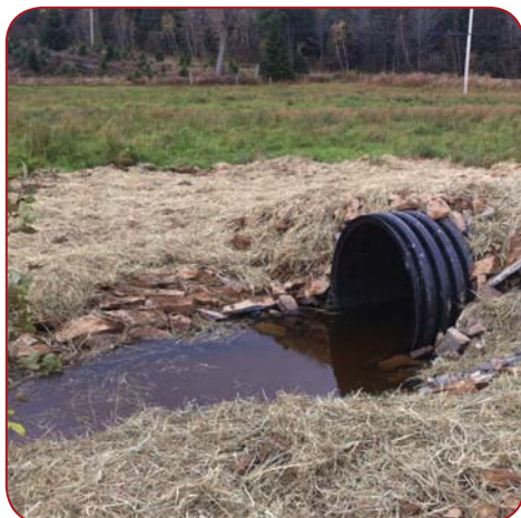
Downstream side of newly installed culvert at DeLong Farm.
