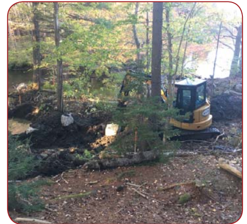
Construction at the Rhodenizer Dam run-around channel.
