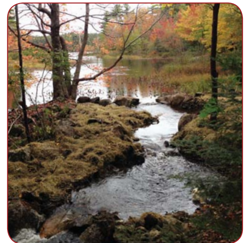
Lake inflow at the completed run-around channel at the Rhodenizer Dam.
