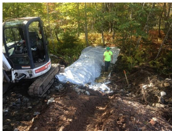
Figure 4: (Left) Dumping load of municipal compost. Figure 5: (Right) Constructing outlet weir in eastern side of restoration site.
